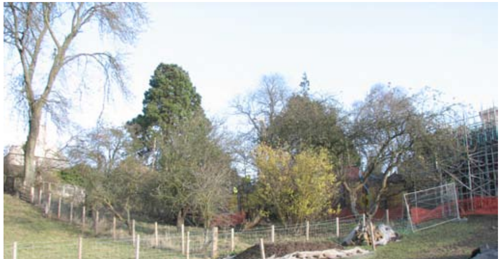
Mount Pleasance orchard; partly damaged by the collapse of the retaining wall supporting the road. Reconstruction works at right of frame.
